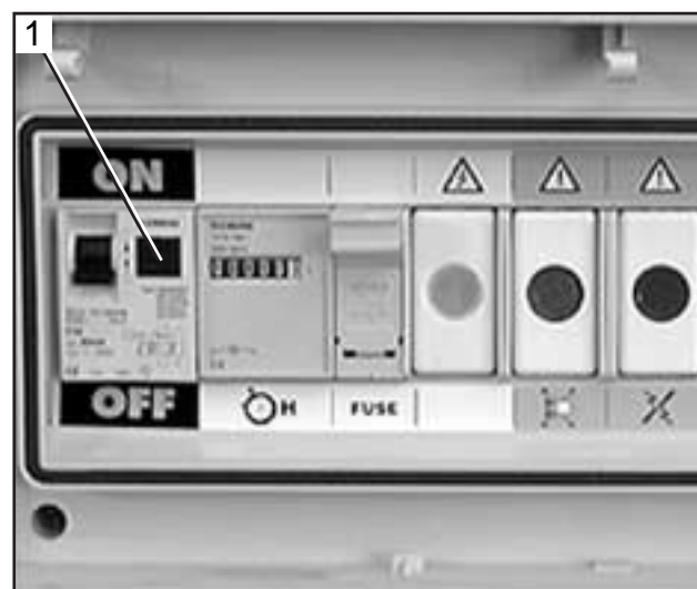
Fig. 50 Fault current circuit breaker
